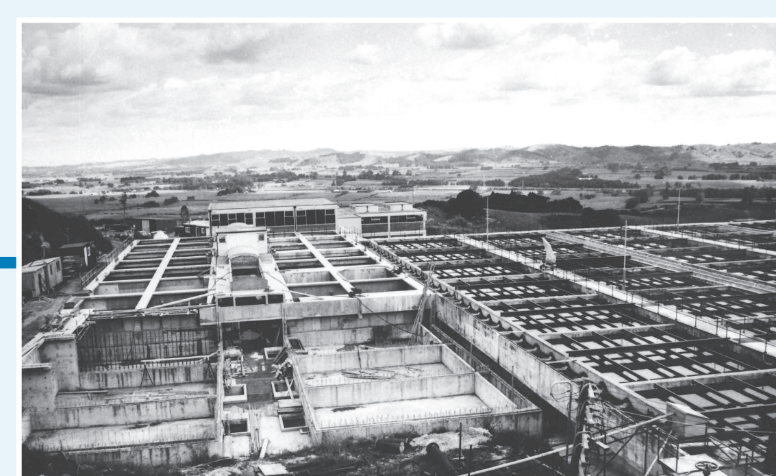
Ardmore Filtration Station during construction
