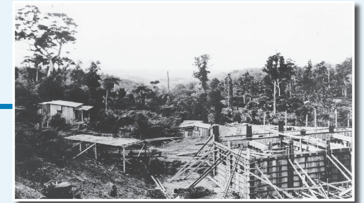
Waitakere Filtration Station during construction
